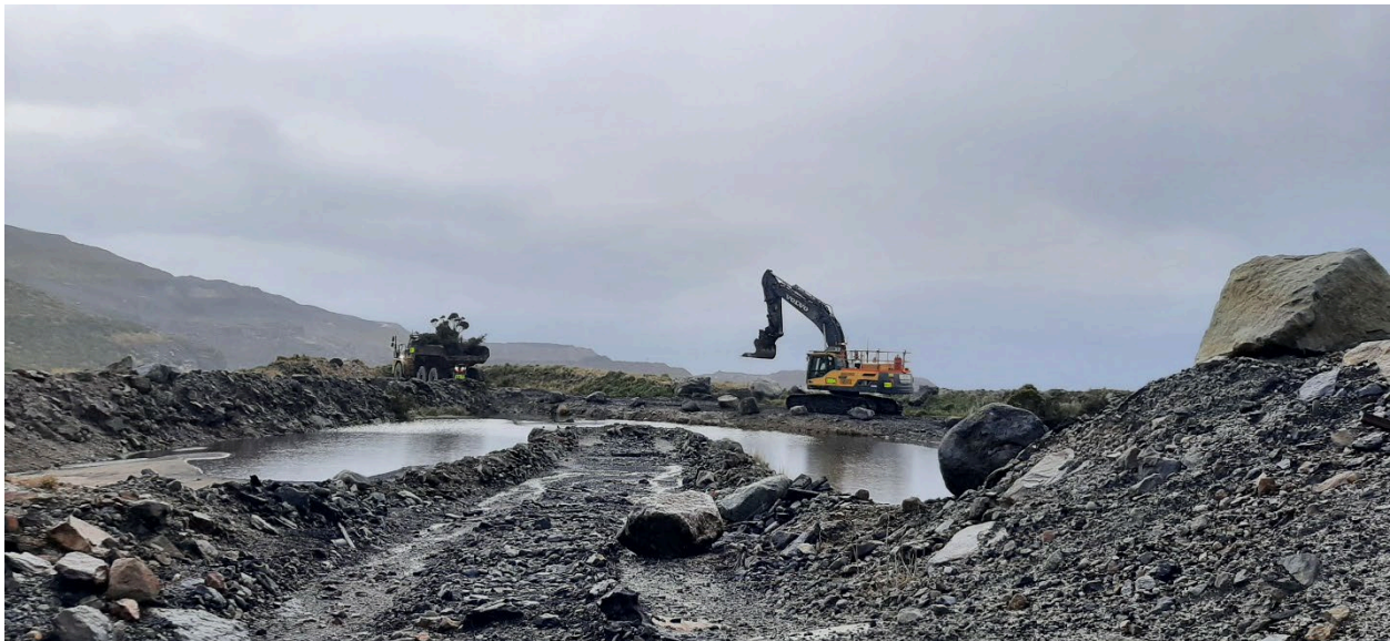
Demonstration of direct vegetation transfer environmental reclamation technique. Vegetation, including a thick layer of original soil and roots, is directly transferred to its new location in a reclaimed area.
